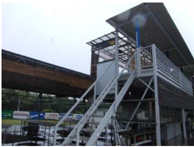
South Gate for down
